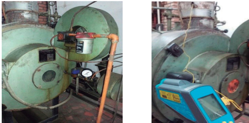
Figure 4. Experimental data collection, Continental F10C boiler Source: the authors.
